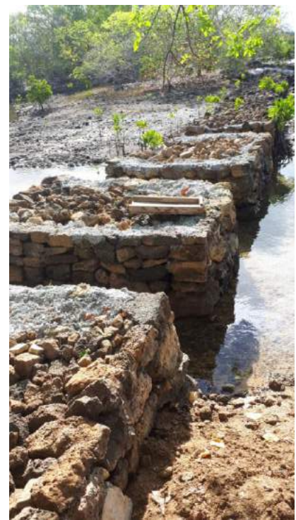
Pictures illustrating the consolidated structures, carried out by two local fishers, facilitating waterways between mangrove ponds in the coastal marine wetland @EPCO / Estelle DEJA.
