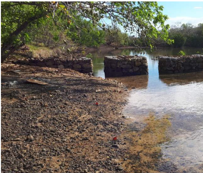
Pictures illustrating the consolidated structures, carried out by two local fishers, facilitating waterways between mangrove ponds in the coastal marine wetland @EPCO / Estelle DEJA.
