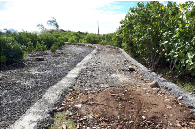
Road consolidation throughout the length of the road by local residents of the Residences la chaux @ EPCO/Estelle Deja
