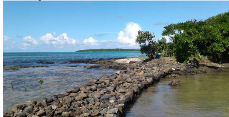
RENOVATED BARACHOIS WALL BY LOCAL RESIDENTS, LA CHAUX, MAURITIUS ©EPCO/ESTELLE DEJA
